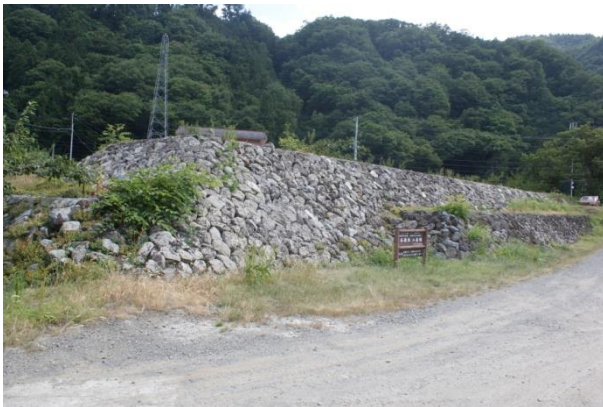
③積石出し二番堤
